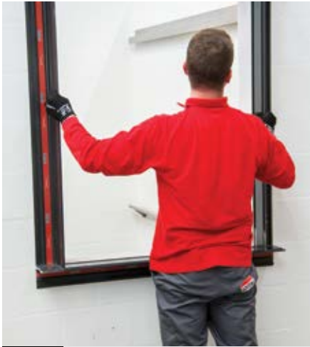
09 Pick up the frame and press it against the wall while moving up and down, left to right
