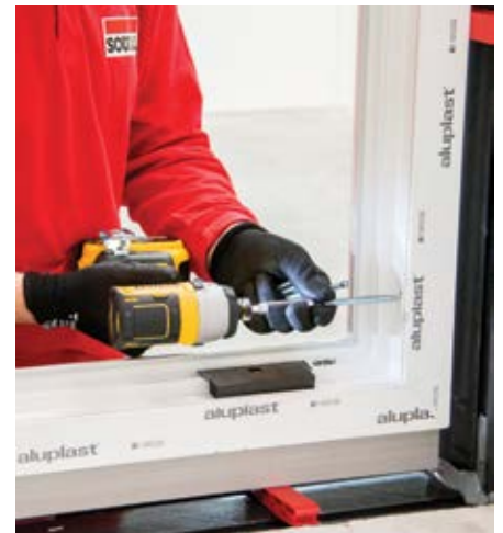
14 Fix the windows mechanically
