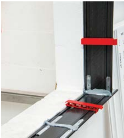
12 Seal the inner corners and position the spring clip
