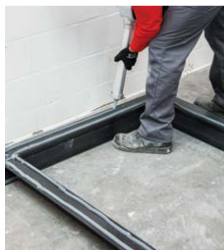
08 Apply the adhesive continuously, in 2 beads, onto the frame
