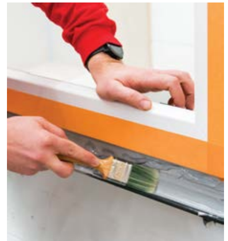
17 Seal with Soudatight Hybrid on the outside
