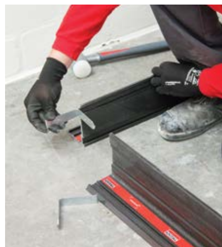
03 Insert the corner connector
