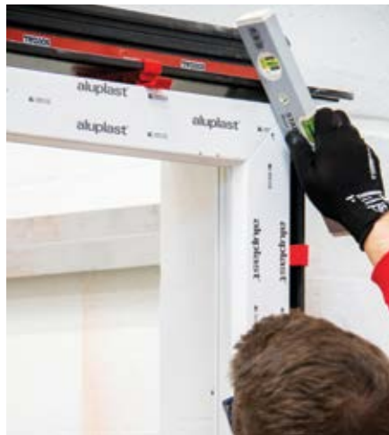
13 Pre-drill the window, insert and align the window
