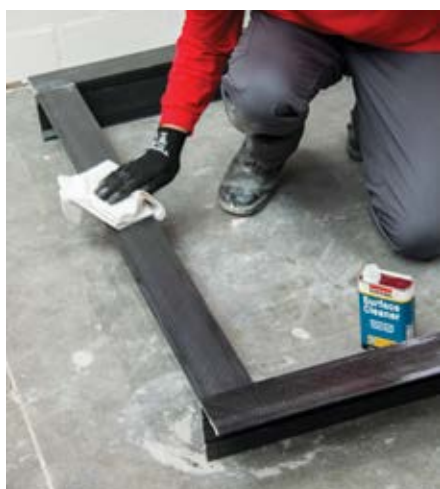
06 Clean the backend of the frame
