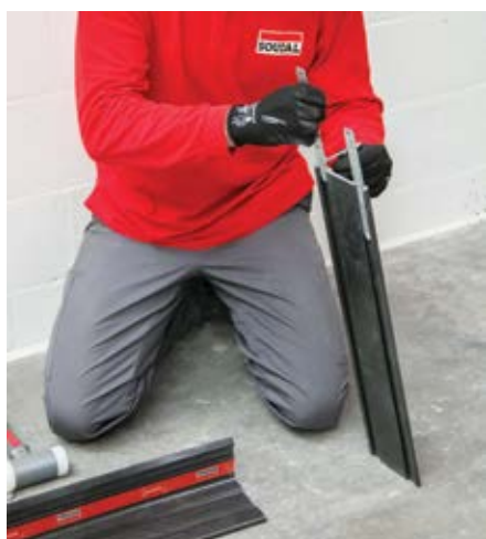
04 Connect 2 frame element or cut-offs with the link connector
